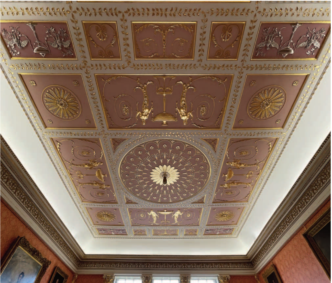
Above, plaster after treatment
